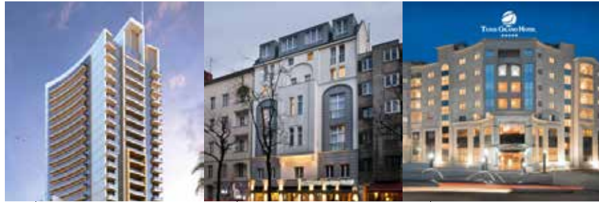
Burj Damac Waterfront Doha Qatar
