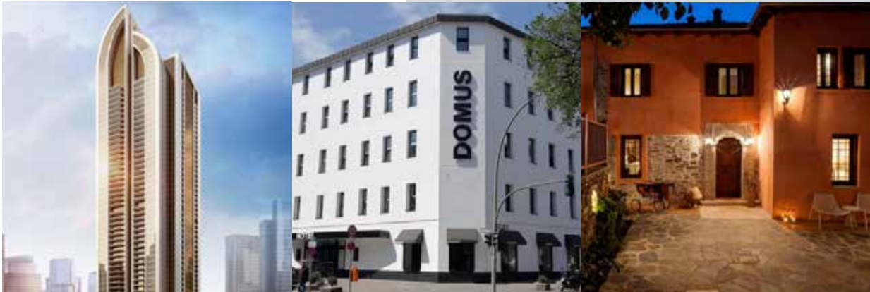
Al Duja Tower Dubai UAE
